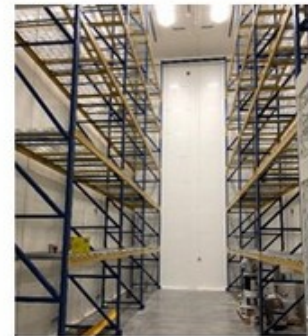
New controlled substance vault expansion
